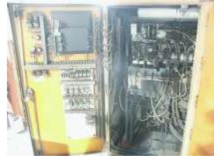
**A control panel door left open to prevent over-heating**
